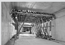
Casseforme per tunnel
