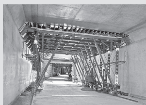
Casseforme per tunnel
