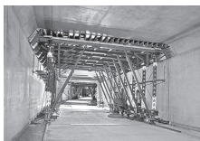
Casseforme per tunnel
