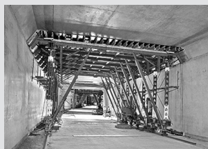
Casseforme per tunnel
