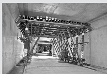
Casseforme per tunnel
