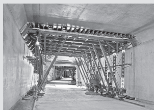
Casseforme per tunnel
