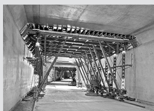
Casseforme per tunnel
