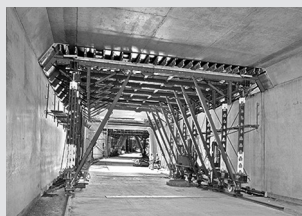
Casseforme per tunnel
