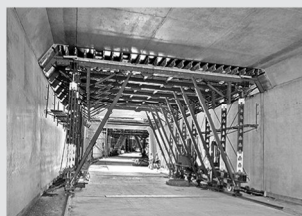
Casseforme per tunnel
