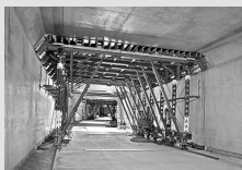
Casseforme per tunnel
