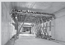
Casseforme per tunnel
