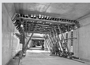
Casseforme per tunnel
