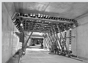
Casseforme per tunnel
